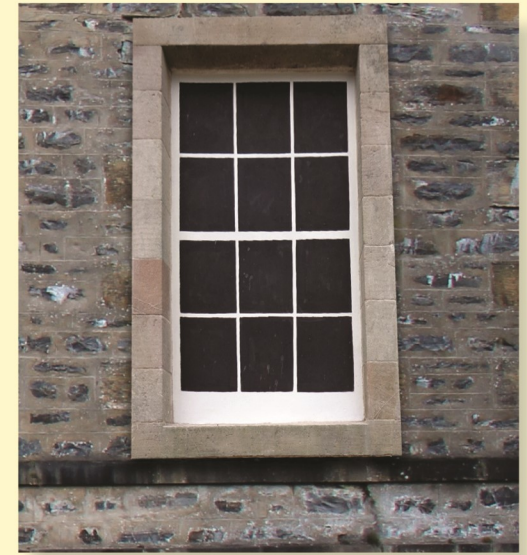
Replacing window glass would be costly and subject to vandalism so all windows will be boarded and painted to simulate windows.
